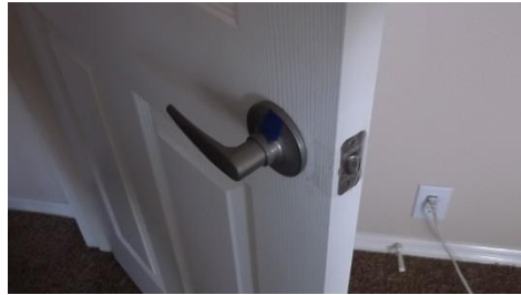
3. Ball latch missing at linen closet downstairs next to master
