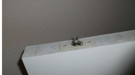
3. Ball latch missing at linen closet downstairs next to master
